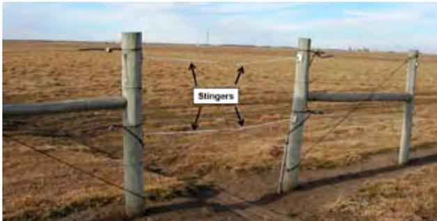
**Figure 6.** Pivot tower gate for a two-wire high-tensile electric fence. *Note:* In this example, insulated wire in conduit is buried beneath the wheel-track to connect both sides of the fence and a wooden plank has been placed in the wheel track to reduce rut development through the gate.
